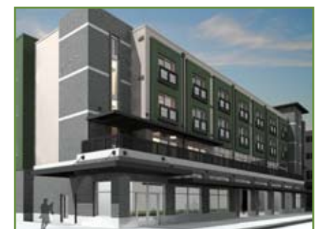
Construction on the Compass Veterans Center - Renton began in September 2009.
