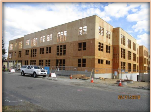
Exterior Walls Level 3
