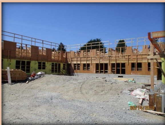
Exterior & Interior Walls Level 2
