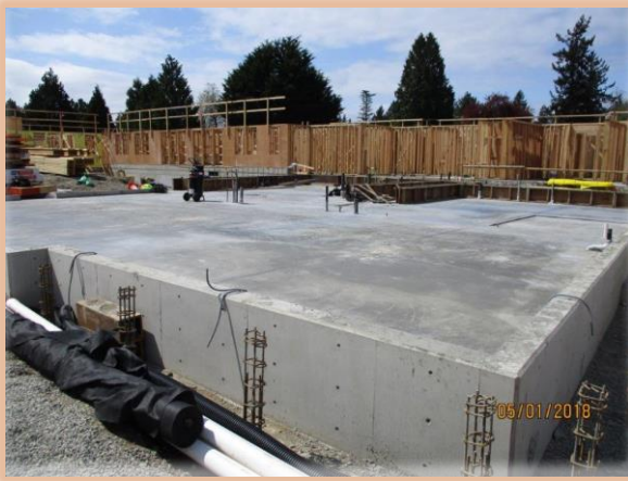
N Slab on Grade & Level 1 Walls
