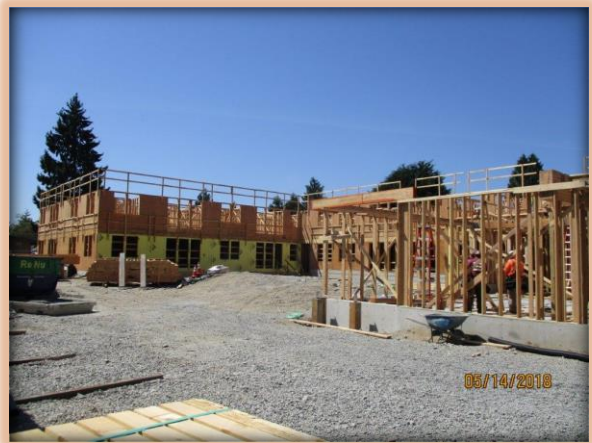
Working on Levels 1 & 2
