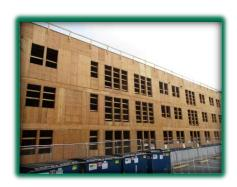
During the upcoming month WALSH will complete the roof, begin weather barrier, windows, siding, and continue installation of plumbing, electrical, HVAC, and fire sprinkler systems.
