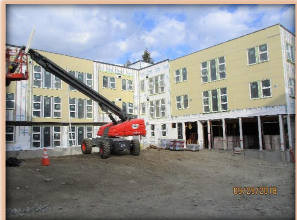
Siding installation - courtyard
